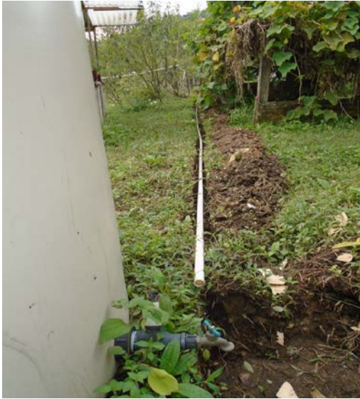
Implementation of irrigation water system
